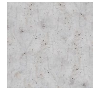
Masonry Concrete Stained
